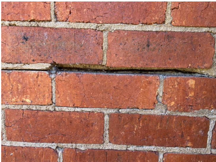
Photo 1: Corrosion to brickwork reinforcing mesh. Two consistent lines around the building.
