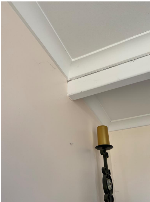
Photo 5: Bearing failure to steel roof support beam. Likely related to termite damage.
