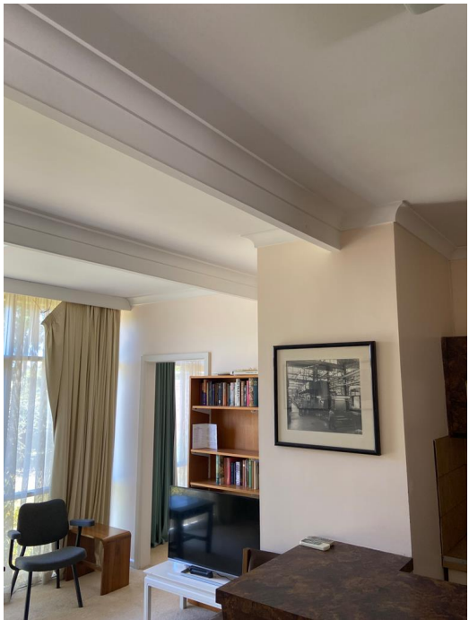
Photo 4: Structural roof beams – different layout to original plans
