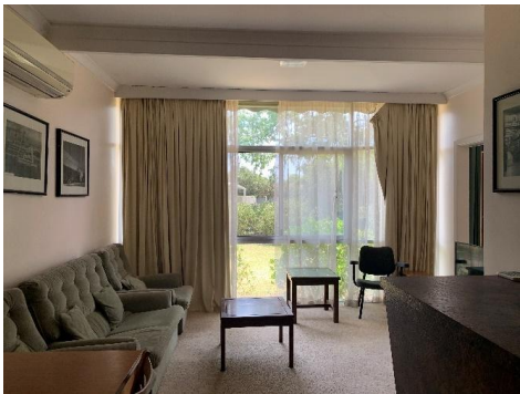
Figure 33. Livingroom area with bowing ceiling beams.
