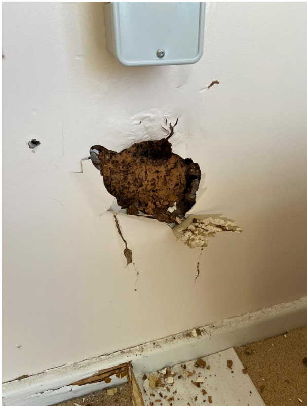
Photo 2: Extensive termite damage throughout.
