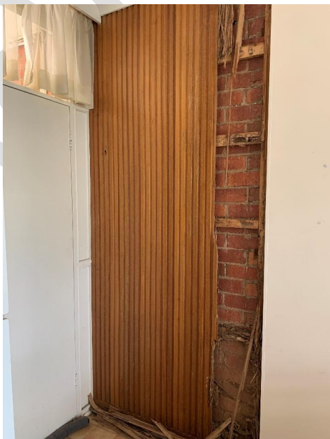
Figure 31. Internal cladding damage behind the front door.
