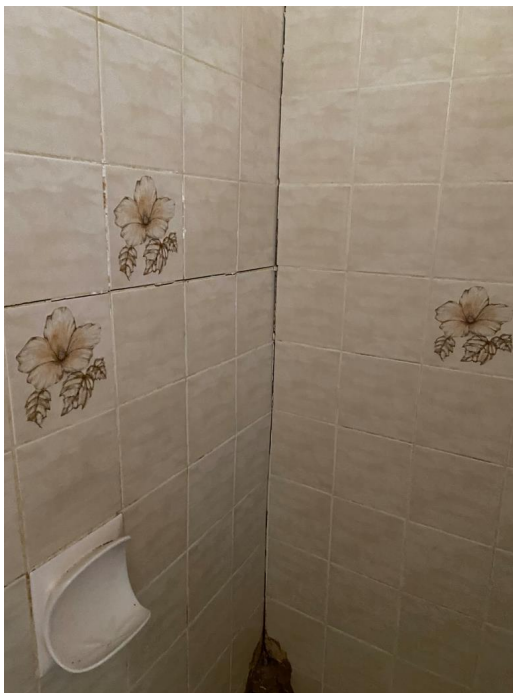
Photo 8: Cracking and evidence of termite damage to wet area walls.
