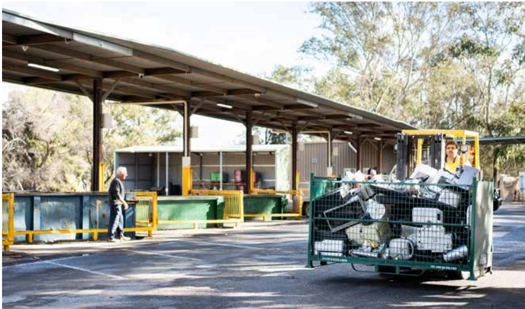
Resource & Recovery Waste Transfer Station
