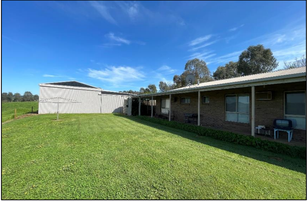
Rear of farm dwelling showing shedding and water tank
