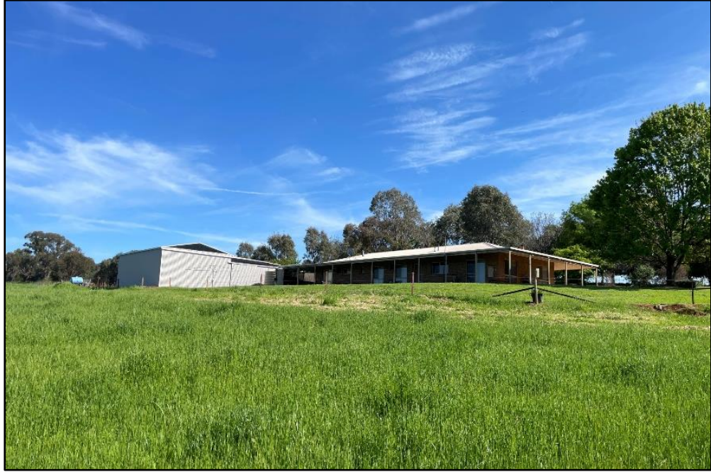
View north to rear of farm dwelling and shed
