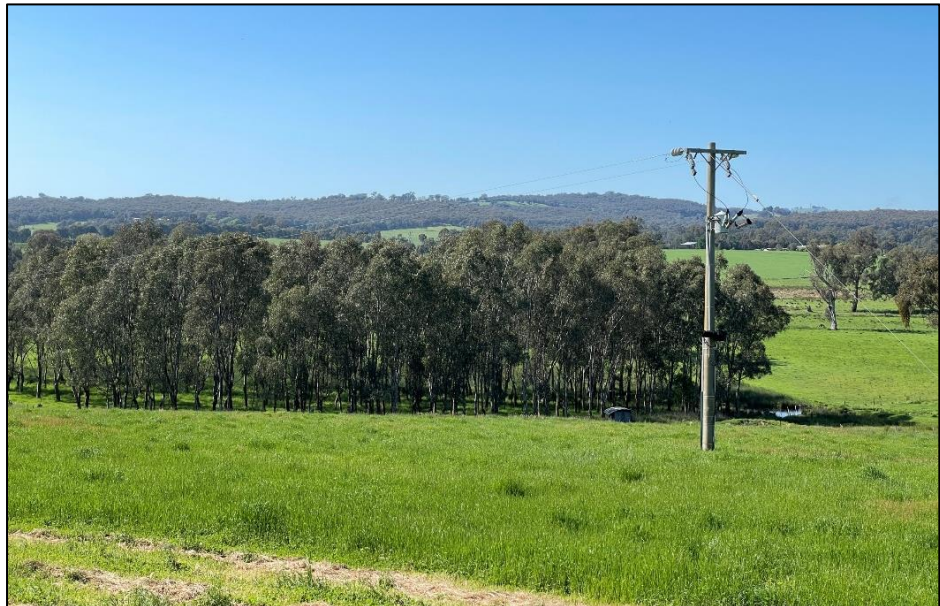
View south to existing pump (for domestic water supply) and overhead powerline
