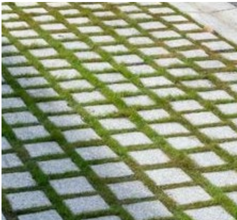
Use of reinforced grassing paving
